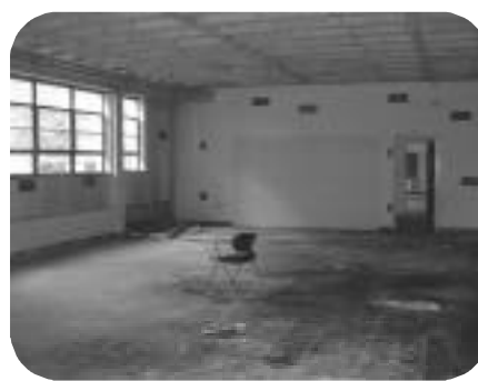
Picture this! Stripped now, this former science lab will house eight of 14 booths.
